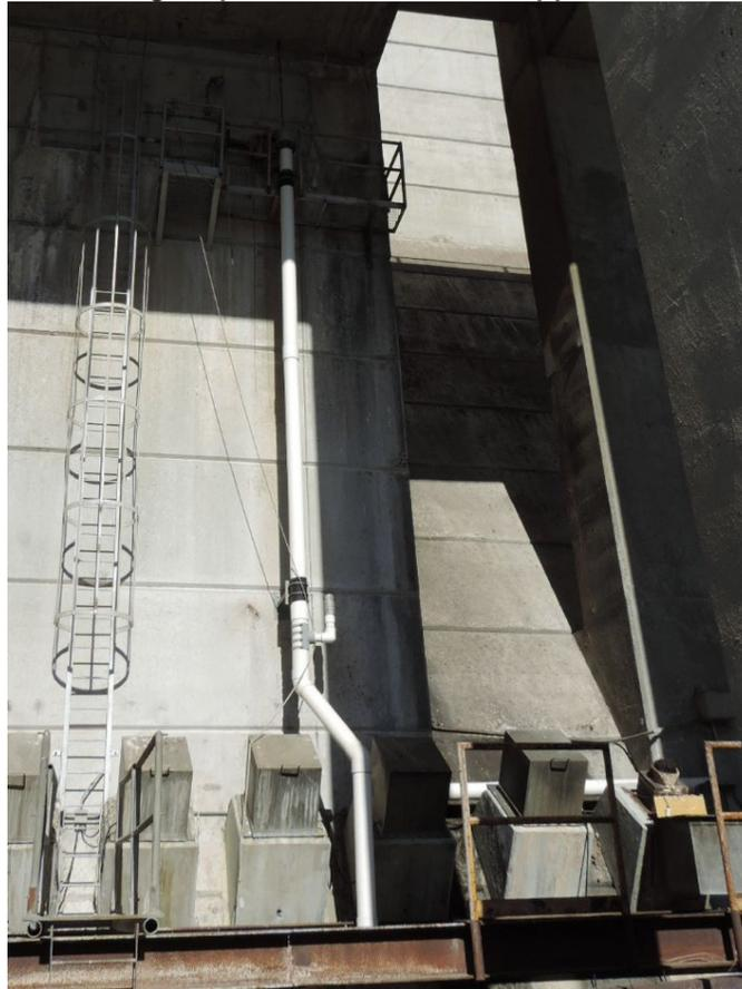
**Figure 3-7. Closer View of the Existing Drain Valve for Diffuser 16.**
